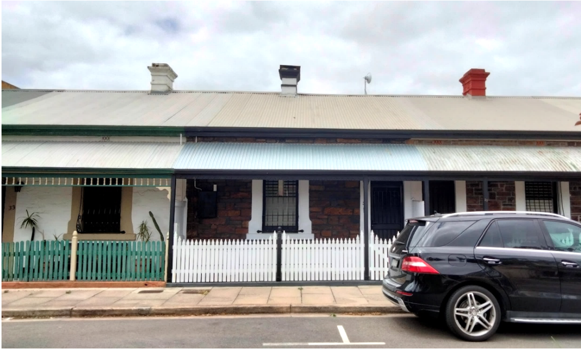
Photo 3.1 - Subject site viewed from McLaren Street
